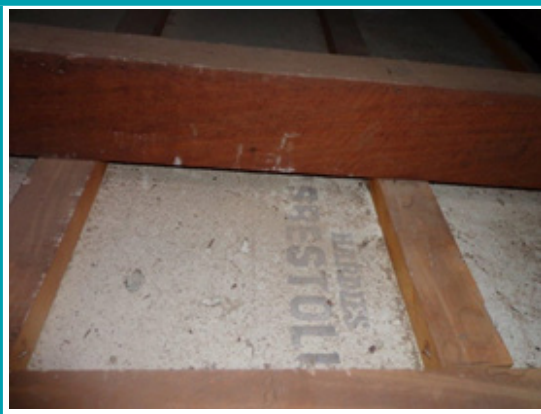
Figure 1 Rear side of LDB ceiling sheet showing trade name
