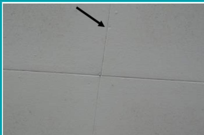
Figure 6 Recessed fastener heads in LDB
